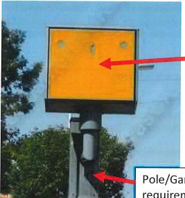
Replace housing with new one that allows digital camera to be inserted. Costs to be borne by local authority.
